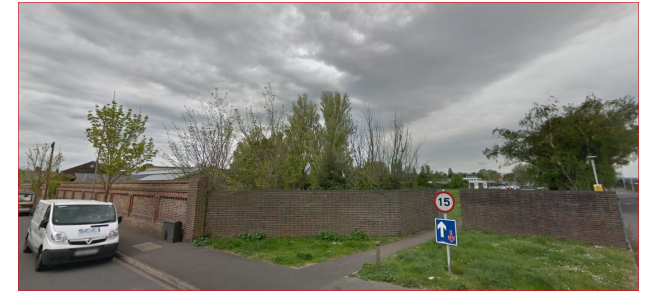
Figure 3b Boundary wall on Locksway Road
