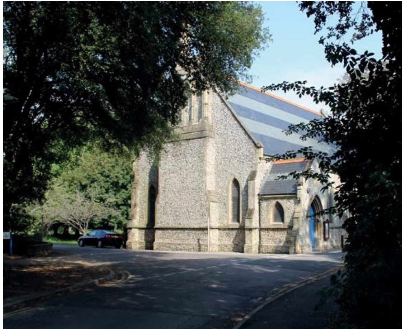
Figure 3. St James Hospital Chapel (East elevation)
